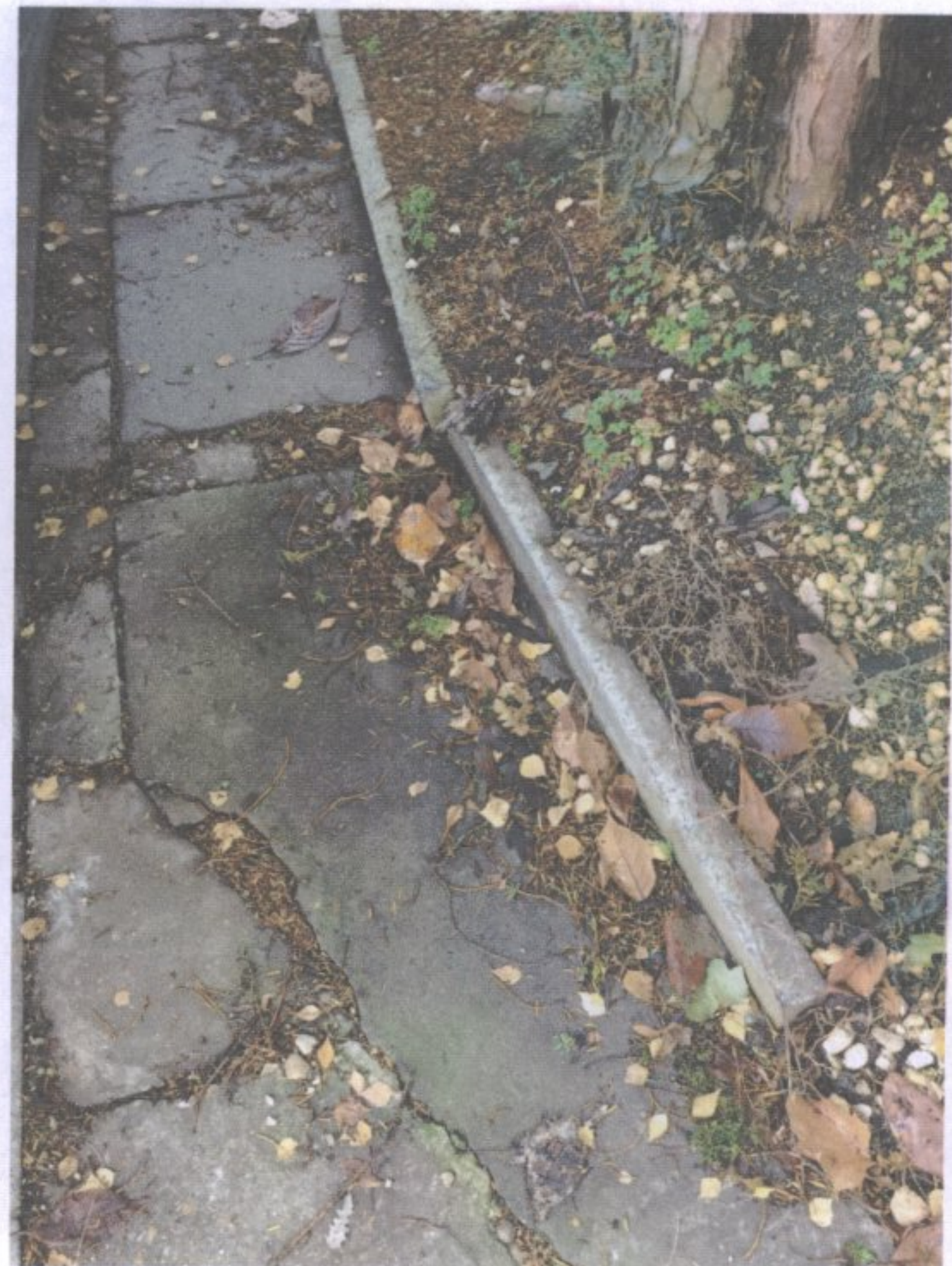
Photo 2: hazardous damage to paving due to expanding root system.
